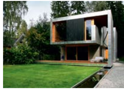
This villa at Smestad outside of Oslo features solid wood elements in the walls and roof supplied by Moelven MassivTre AS. The architect is Knut Hjeltnes AS Sivilarkitekter MNAS.
