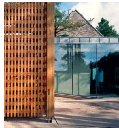
The load-bearing structures at Mortensrud Church are made of glulam.
