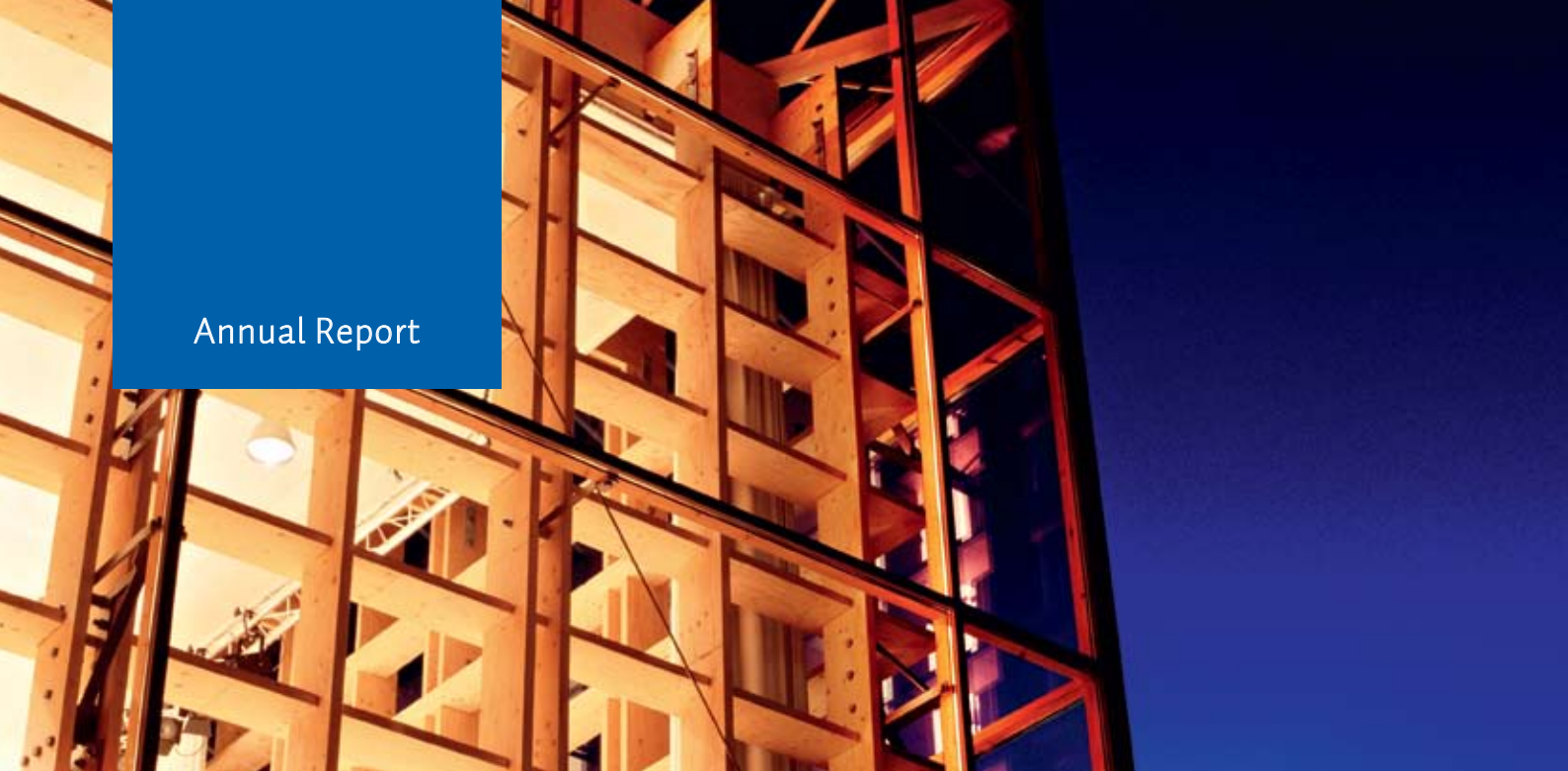
Kerto beams supplied by Moelven are clearly visible at the cultural and recreational centre at Jemtelandsgade in Copenhagen.
