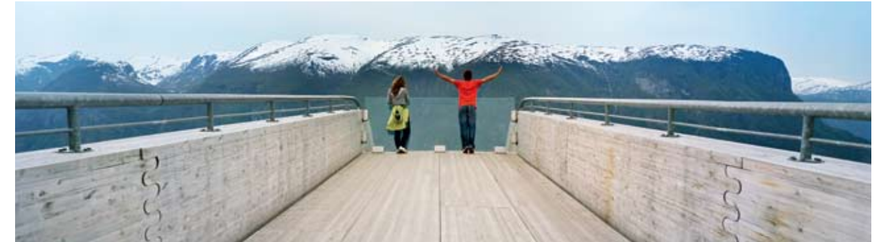
The viewing station at Aurland fjord, Stegastein, was built using glulam from Moelven and has attracted international attention.
