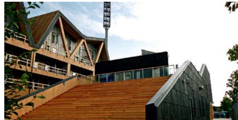
Egenes Park in Stavanger consists of 56 apartments, a daycare centre for children and several other buildings and is one of the Nordic countries' largest construction projects in solid wood. Moelven MassivTre AS and Moelven Limtre AS supplied the load-bearing structures, as well as building elements for the floor, walls and roof.
