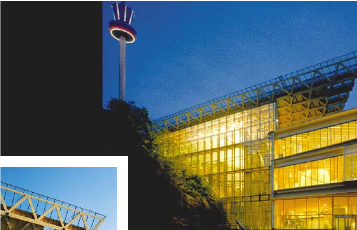
Glulam structures in the Universeum in Gothenburg.
