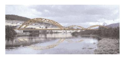
other examples of the great potential glulam has compared to steel and concrete. Moelven has also, in collaboration with the Norwegian Highways Department, developed a concept for building timber bridges.
