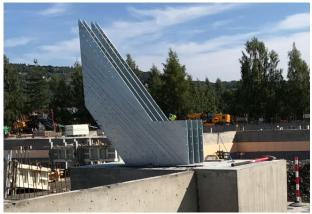
Figure 15: Base connection of the corner column and diagonal.
