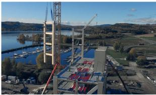
Figure 16: Hoisting of frames.
