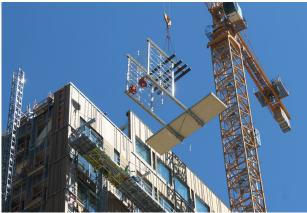
Figure 17: Hoisting of balconies with tower crane.
